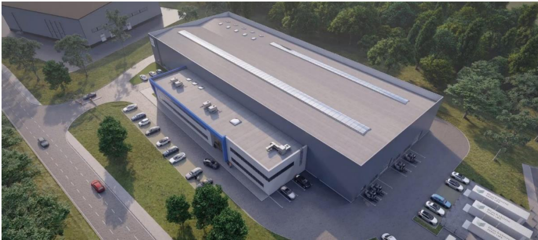
Blackstone Technology GmbH in Döbeln, Germany
